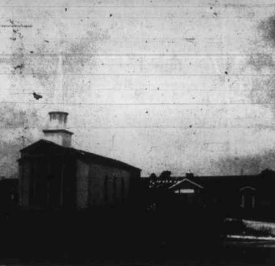
Work is expected to be completed before the end of the year on this beautiful new church and educational facility for the United Methodist Church in Eagle Lake.
